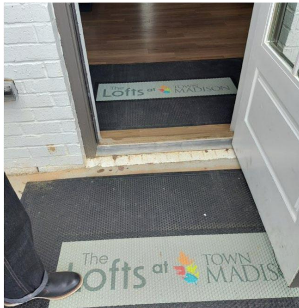
Figure 1: Exterior Threshold at Building Entrance
