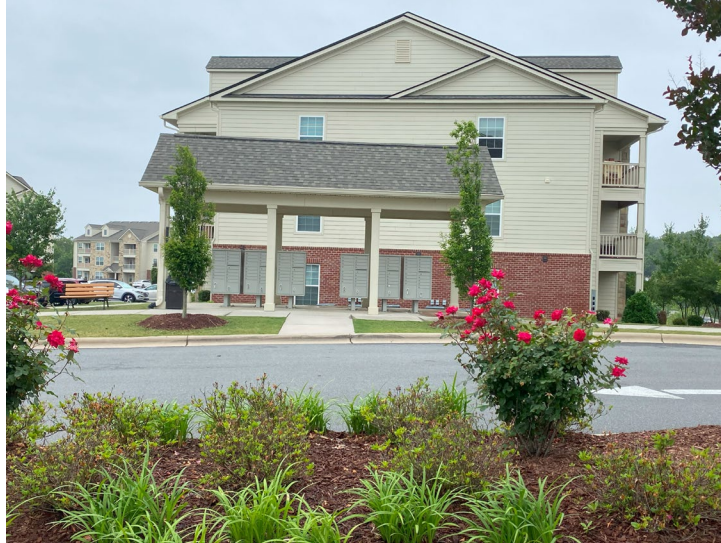
Figure 18: The route to the mail kiosk by the first gate at Revere at Tega Cay does not have curb cut.
