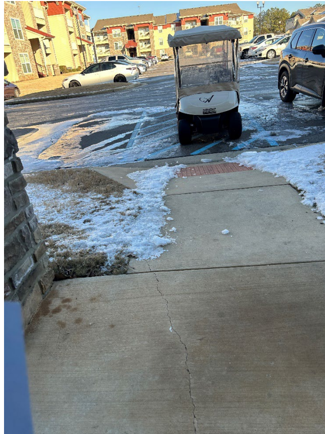
Figure 16: Property vehicle blocking accessible route into Building 28
