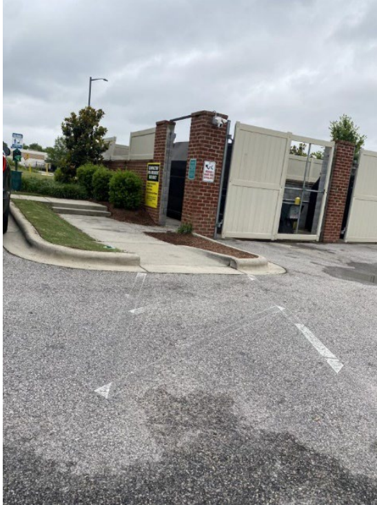
Figure 29: There are no accessible parking spaces for the trash compactor at Revere at Tega Cay. The closest accessible parking space is at Building 12. The accessible route from accessible parking at Building 12 would require descending stairs to the compactor or would require a person with a disability to cross the roadway, where an accessible route has not been maintained because there is no painted crosswalk.
