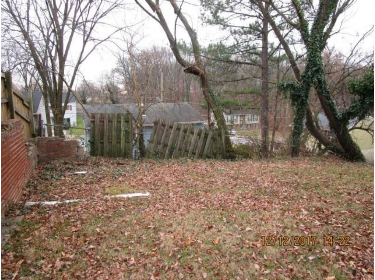
Capitol Heights, MD – Dead leaves and damaged fence
