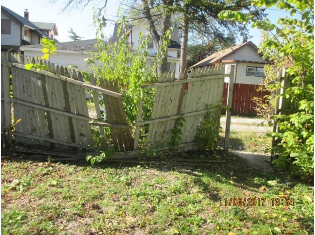
Maywood, IL – Overgrown shrub and damaged fence
