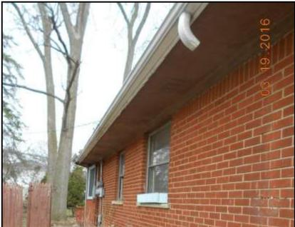
Multiple gutters on this home are either misplaced, broken, or missing all together.
