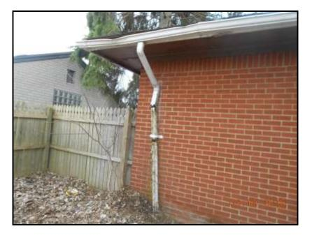
There is a open pipe spilling out water – it is sitting around the home's foundation as well as flowing into the foundation itself.
